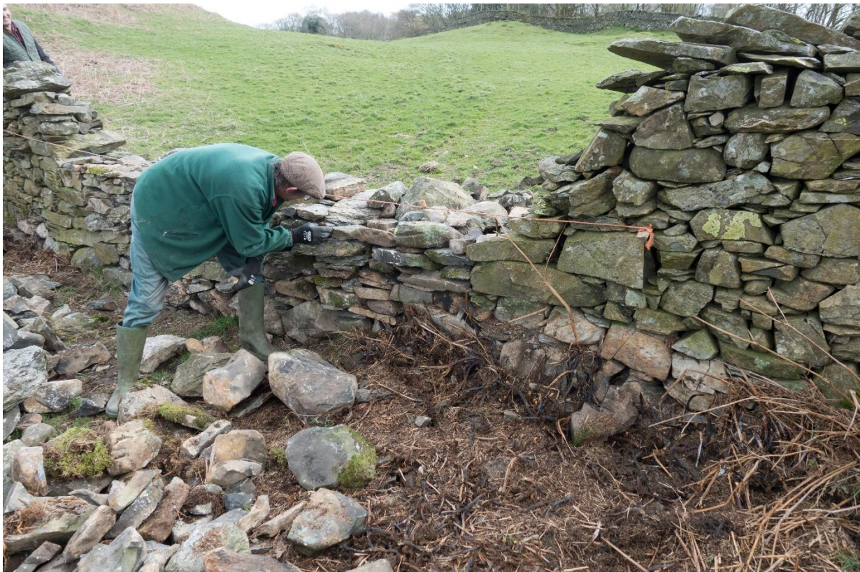
Dry-stone walling in action
